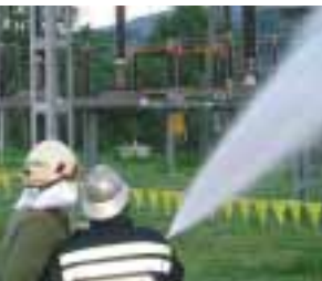
The spraying of live lines and installations with water must be practiced. EVN carries out regular training with fire-fighters for this purpose.
