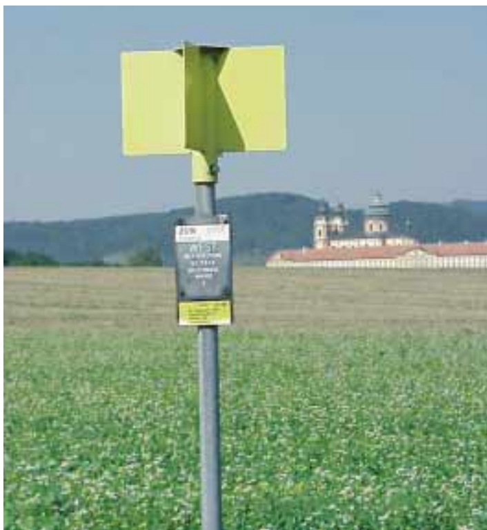
Following recultivation, the only sign of a high-pressure gas pipeline are the markers (see photo).
