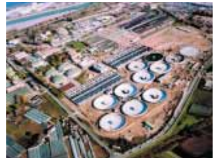
WTE is acting as the general planner for the refurbishment of the central Vienna wastewater treatment plant, which serves 4 million people.
