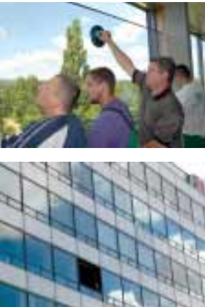
The replacement of the windows at EVN headquarters has provided major energy savings.
