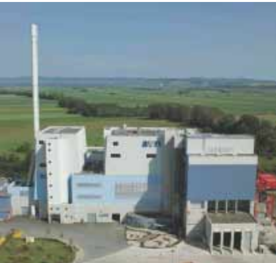
The new AVN waste incineration plant.
