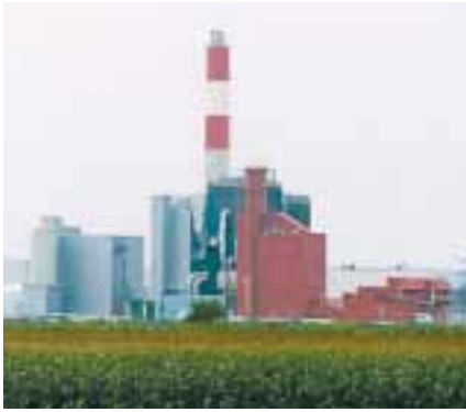
Additional output and efficiency optimisation at Theiss power station during full load operation.
