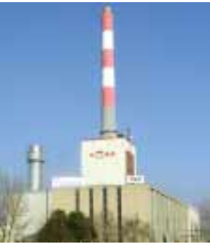
The preparations for accreditation in line with EMAS and ISO 14001 at the Korneuburg power station are progressing at speed.
