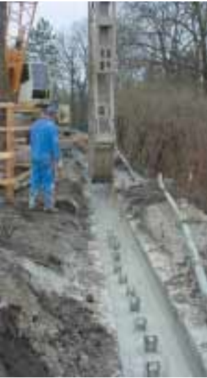
EVN is decontaminating and securing former town gas production sites.
