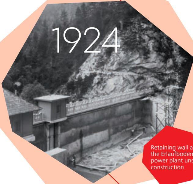
Retaining wall at the Erlaufboden power plant under construction
