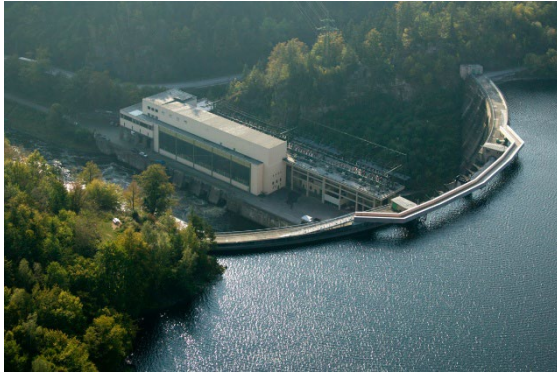
Pumped hydro storage 78 MW installed capacity
