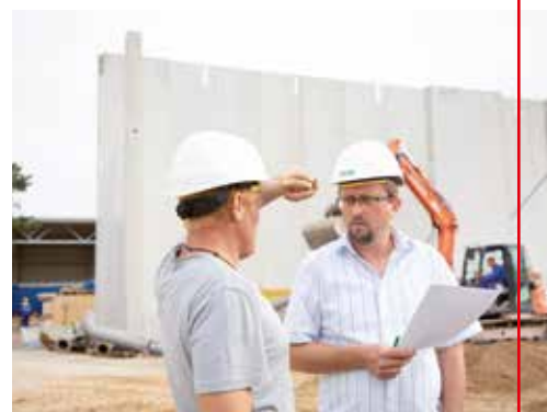
Construction of a biomass heating plant in Klosterneuburg
