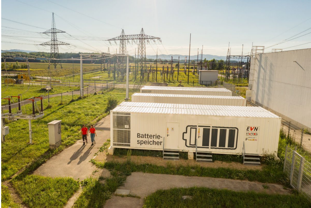
5 MW battery storage pilot plant in Theiss
